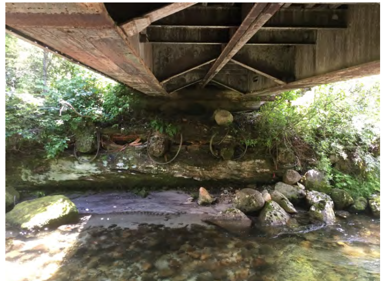
Right Bank Abutment when facing downstream
