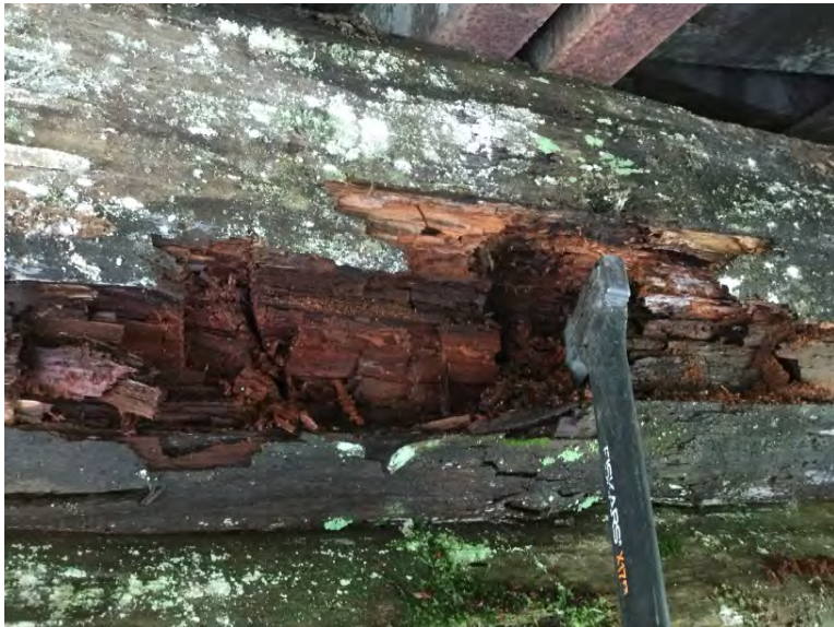
Top face log condition at center left abutment
