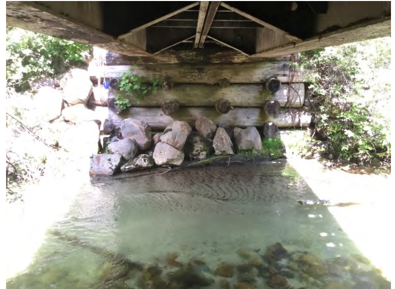
Left Bank Abutment when facing downstream
