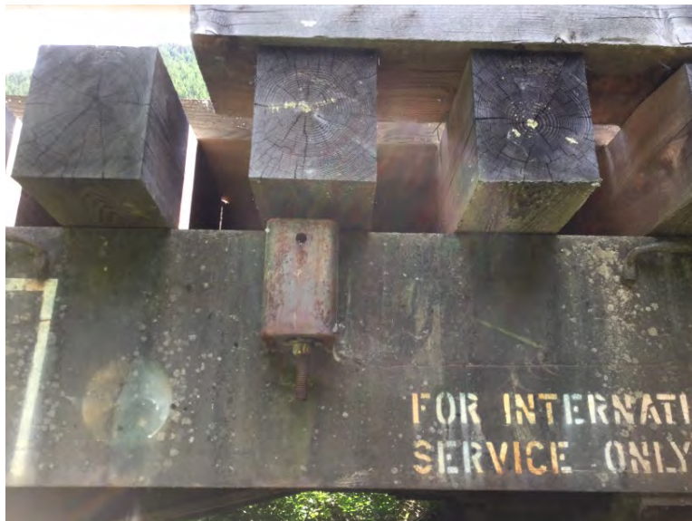
Deck fasteners
